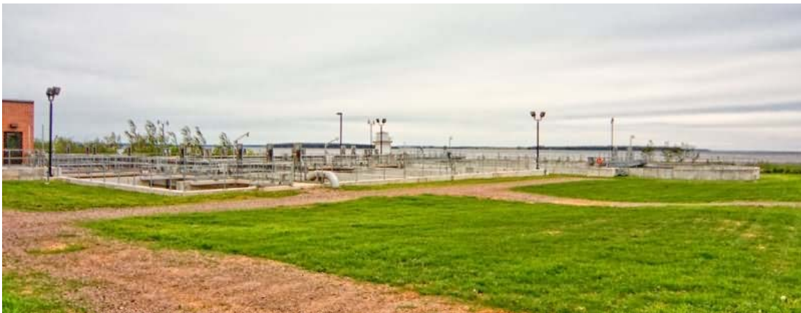
Figure #2 Widescreen of Biological Nutrient Removal System.
